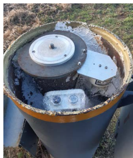
Fig. 2. Pillar one of the geodetic baseline Košice
