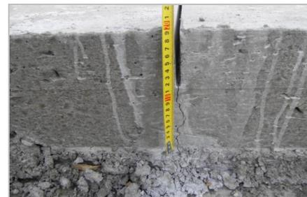
Fig. 9. Form of crack in contraction joints of concrete pavement
