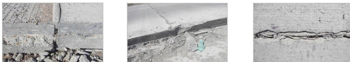
Fig. 11. Contraction joints and expansion joints damaged by slab behavior
