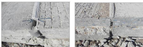
Fig. 10. Measurement of the behavior and length of expansion of horizontally expanded joints
