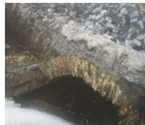
Fig. 3. Sewers built of clinker brick in Kyiv
