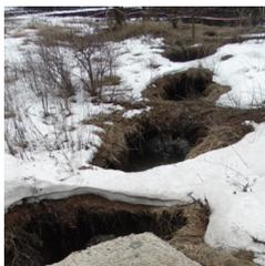
Fig. 1. Sewer deterioration in the area of the Kharkiv Tractor Plant due to biogenic corrosion
