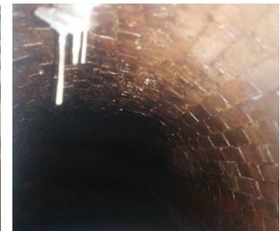
Fig. 4. Sewers built of clinker brick in Kharkiv
